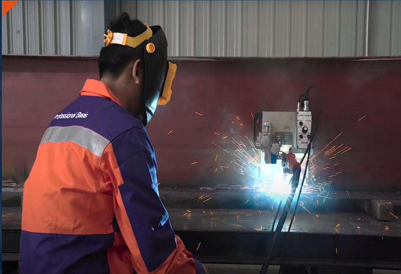
FCAW Semiautomatic Welding
